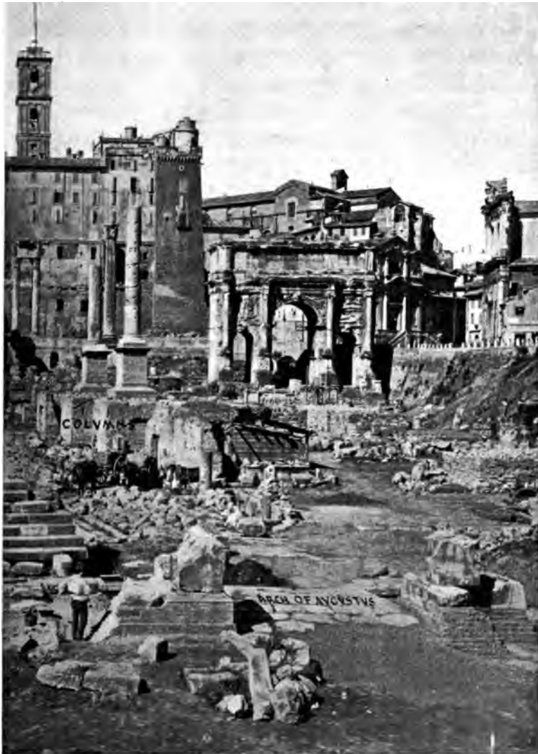
THE REMAINS OF THE ARCH OF AUGUSTUS
